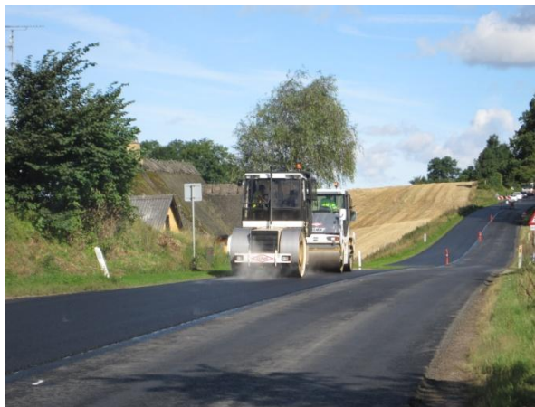
Figure 12 - Construction of Noise Reducing Thin Layers (Denmark)
