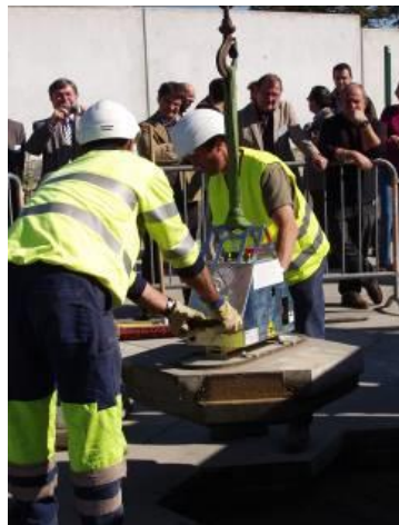
Figure 11 - Laying of Removable Pavement (France)
