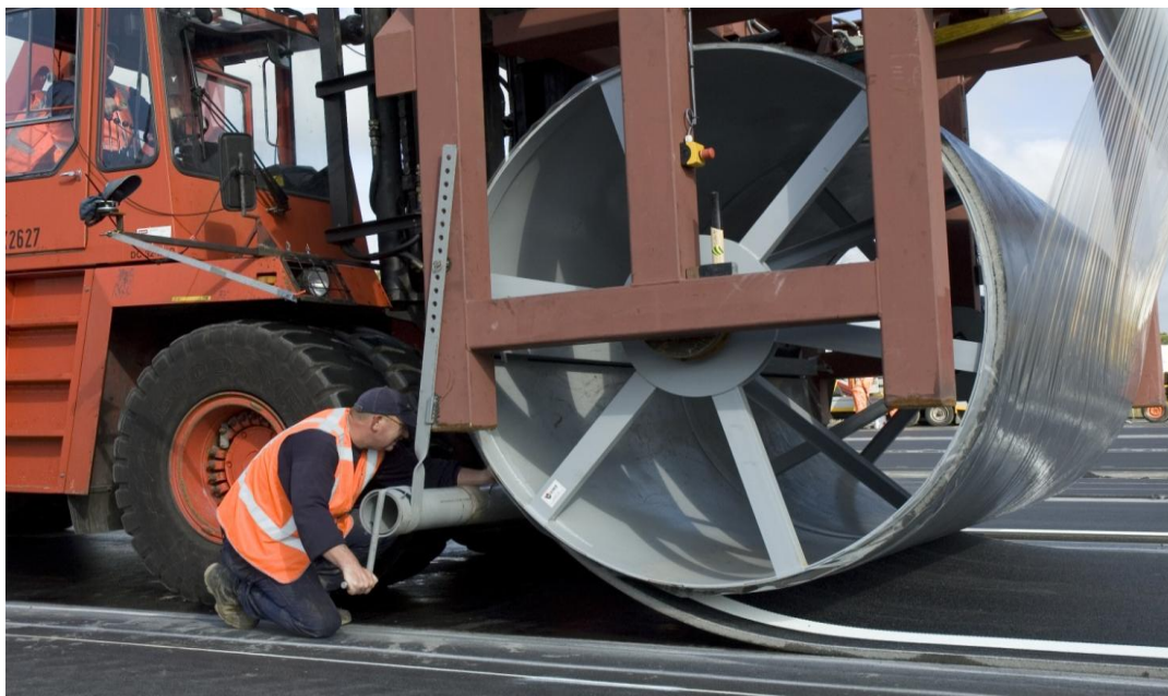
Figure 7 - Rollpave Test Section
