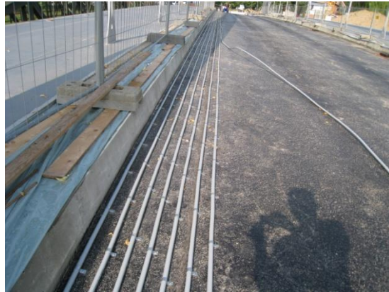
Figure 10 - Laying of bridge deck heating pipes (Germany)
